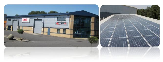
The installation is a 115 No panel, 29.28kW Solar Photovoltaic system using 250W and 260W Znshine monocrystalline panels mounted on a Renusol MetaSol mounting system fixed to a metal trapezoidal roof, and SMA Sunnyboy Inverters. An SMA GA-500 Large Display is displayed in Reception which shows a summary of the energy being produced and the CO<sup>2</sup> being saved.
